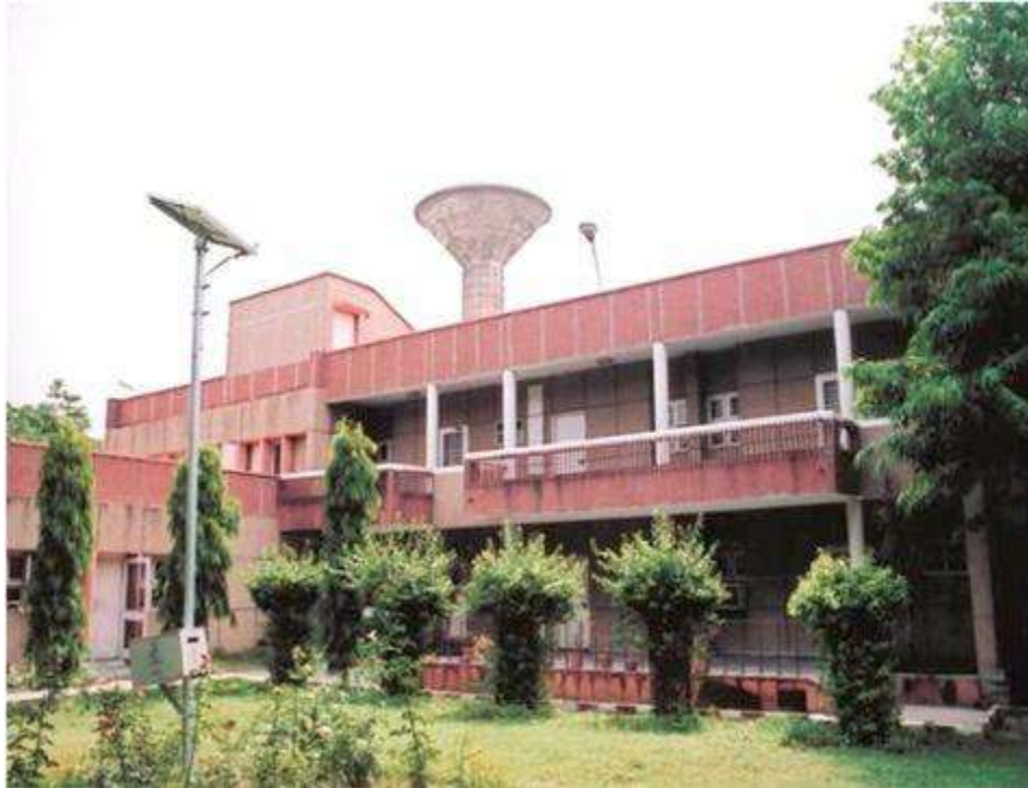
Guest House (8 Double Bedded Rooms)
