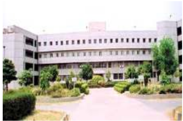
Mechanical Engineering Block
